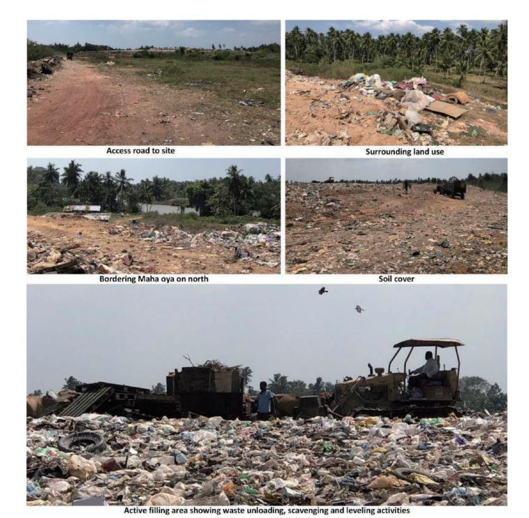
Figure 5-4: Waste discharge and management practices of Ovitiyawatta dumpsite, Negombo MC
